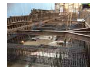
Cừ larsen Sheeting pile
